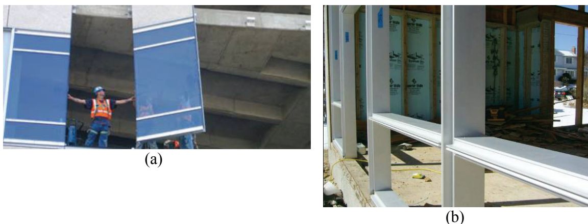
Figure 85: (a) Picture showing the installment of a unitized CW system ( www.sierraglass.com ) and (b) picture showing the construction of the framing for a stick-built CW system ( www.livemodern.com ).
