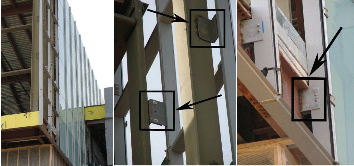
Figure 12: Curtain wall system under construction in State College (Pennsylvania) with connection elements between CW frame and structural frame highlighted.
