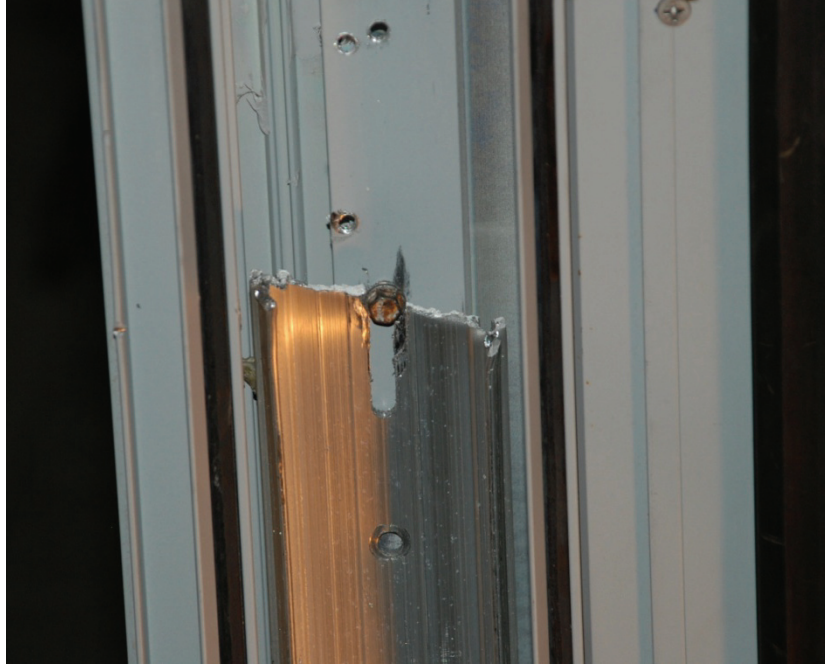
Figure 63: Sheared Boundary Element.
