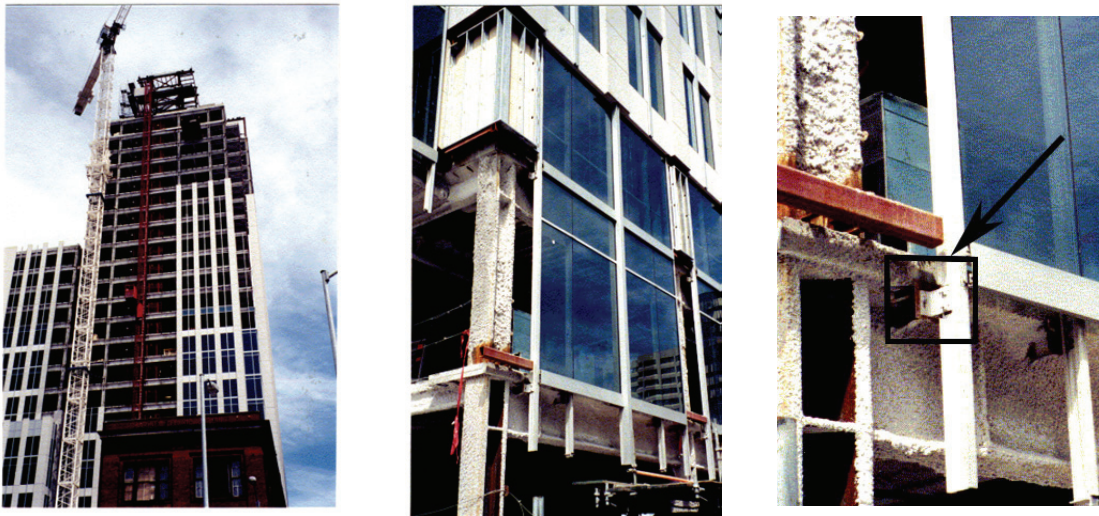
Figure 11: Curtain wall under construction in San Francisco with connection elements between CW frame and structural building frame highlighted.
