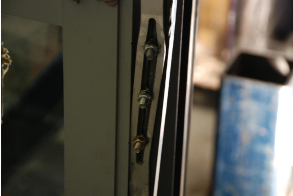
Figure 60: Widening of Slotted-Holes.
