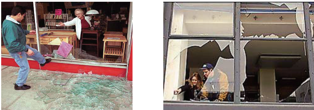
Figure 1: Glass failures documented during the 6.8 M Nisqually earthquake. Photo by Tom Reese/ Seattle Times March 2001.
